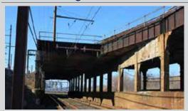
The Sawtooth Bridge carries the NEC over the NJ TRANSIT Morristown Line and the PATH rail line. The bridge is in a state of serious distress and is well beyond possibility of rehabilitation.
