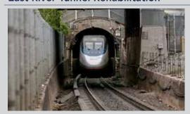
The East River Tunnel consists of four tubes that connect Manhattan to Long Island and are used for Amtrak and MTA Long Island Rail Road services. The tubes, constructed in 1909, require significant upgrades and rehabilitation in order to achieve a state of good repair.
