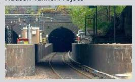
Every weekday, almost 200,000 Amtrak and NJ TRANSIT passengers use the Hudson River Tunnel—originally built in 1910—to travel between New Jersey and Manhattan. The tunnel was significantly damaged by Superstorm Sandy in 2012. While operationally safe, the tunnel today continues to deteriorate due to corrosive minerals that damaged the bench walls, embedded steel, track, and signaling and electrical components.
