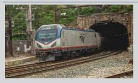
The Baltimore & Potomac Tunnel, built in 1873, runs underneath central Baltimore City and is a key chokepoint on the Corridor. The B&P Tunnel underwent rehabilitation in the 1980s, but that effort was not intended to be a permanent fix. The tunnel requires ongoing maintenance. High saturation of water in the soil beneath the tunnel causes its aging floor slabs to sink, forcing Amtrak to make repeated repairs.
