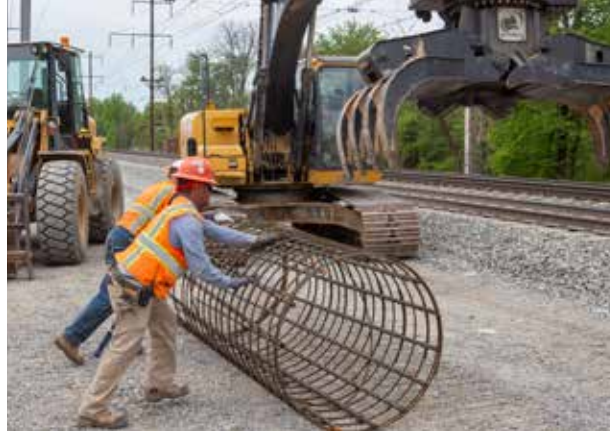
Left: Hanson Interlocking near New Carrollton, MD. Middle: Crews installed new catenary foundations in 2019. Right: A new central instrument house is raised off the ground to protect the interior electronic equipment from potential flooding.
