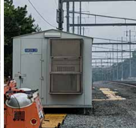
Left: Hanson Interlocking near New Carrollton, MD. Middle: Crews installed new catenary foundations in 2019. Right: A new central instrument house is raised off the ground to protect the interior electronic equipment from potential flooding.
