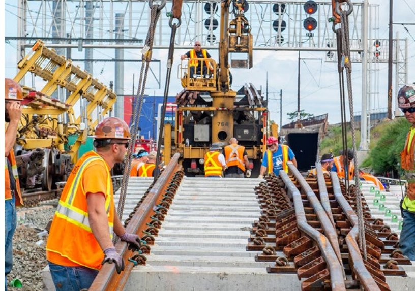
Above left: President Joe Biden speaks at an April 2021 event in Philadelphia, PA celebrating Amtrak's 50th anniversary. Above right: MTA Long Island Rail Road crews install new track at Harold Interlocking in Queens, NY.
