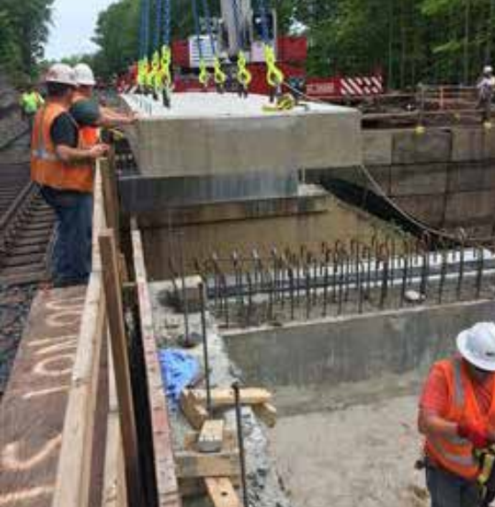
Left: Workers replace sections of Batchelder Road Bridge as part of the CT rail Hartford Line Program. (Source: NHHS Rail Program). Right: The Baltimore & Potomac Tunnel was built in 1873 and is a key chokepoint in the NEC since the right-of-way is reduced from four to two tracks and poor condition require trains to reduce speeds to 30 mph. (Source: Amtrak).
