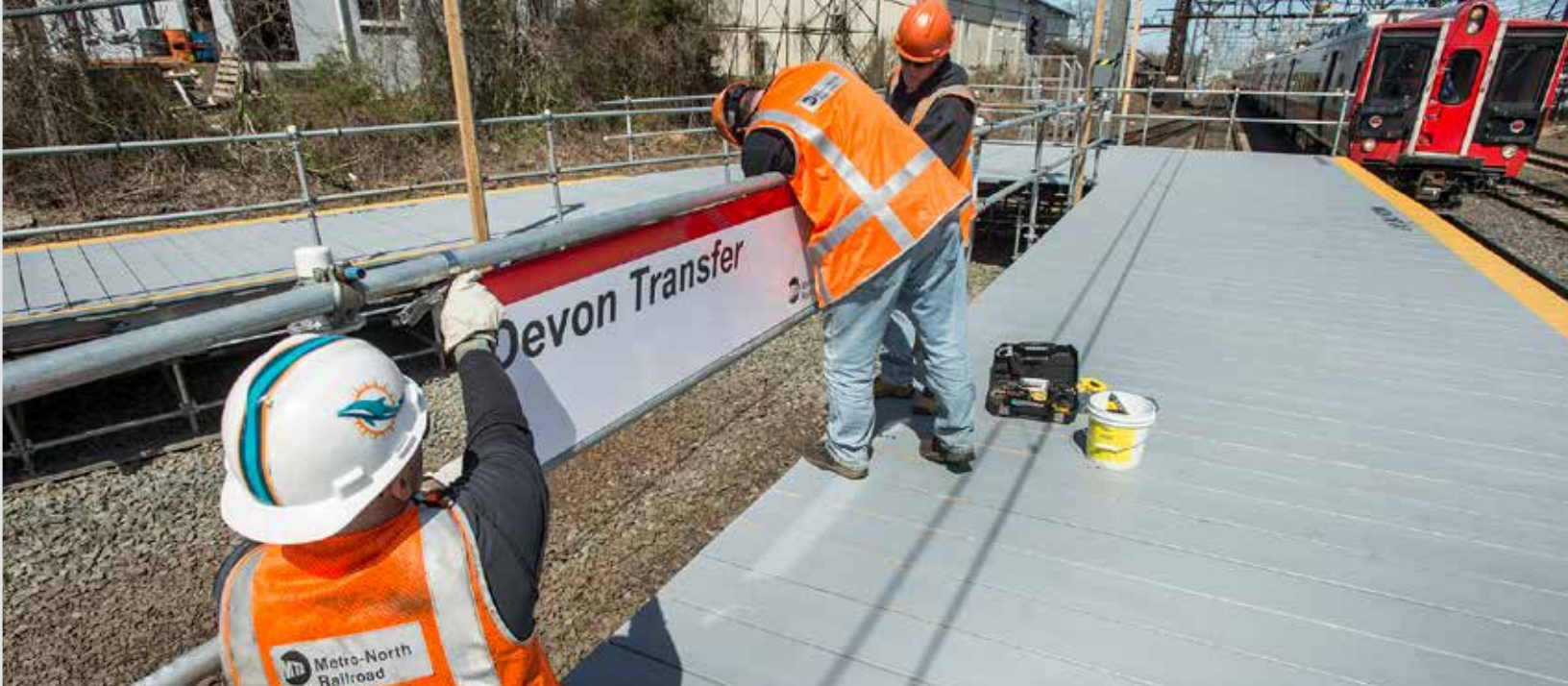
Metro-North workers install a temporary platform on the New Haven Line. Source: NY Metropolitan Transportation Authority.
