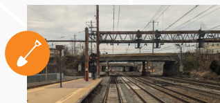
Mid-Atlantic South Signal System Upgrades
