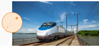
Bush River Bridge Replacement Program
