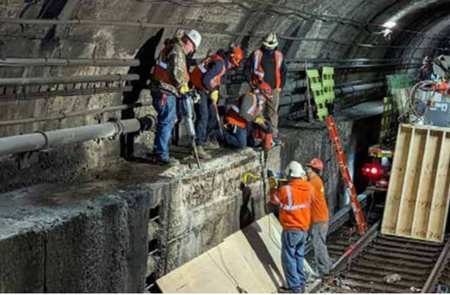
Above left: Amtrak workforces prepare the North River Tunnel benchwall for new concrete to be poured as a part of ongoing interim reliability improvements (NJ/NY). Above right: Track and signal upgrades at Tower 1 and Cove Interlockings will address reliability and resiliency issues near Boston South Station (MA).
