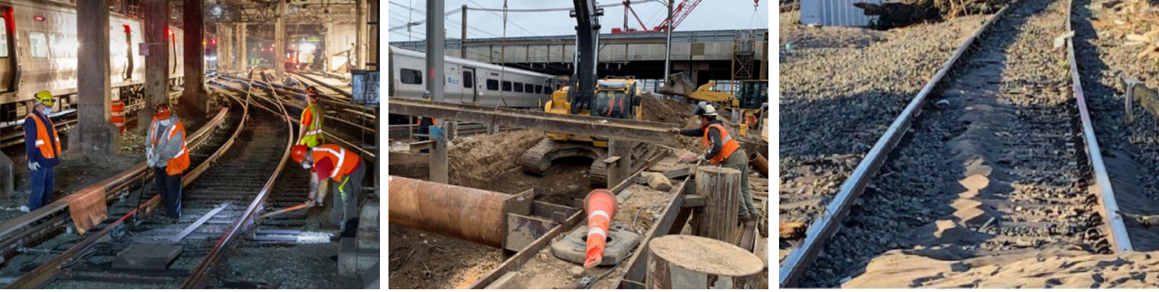
Above: The capital renewal of basic infrastructure includes the routine repair or replacement of existing basic infrastructure assets, to keep the NEC safe for train operations. Investments in track assets have steadily grown year-over-year.
