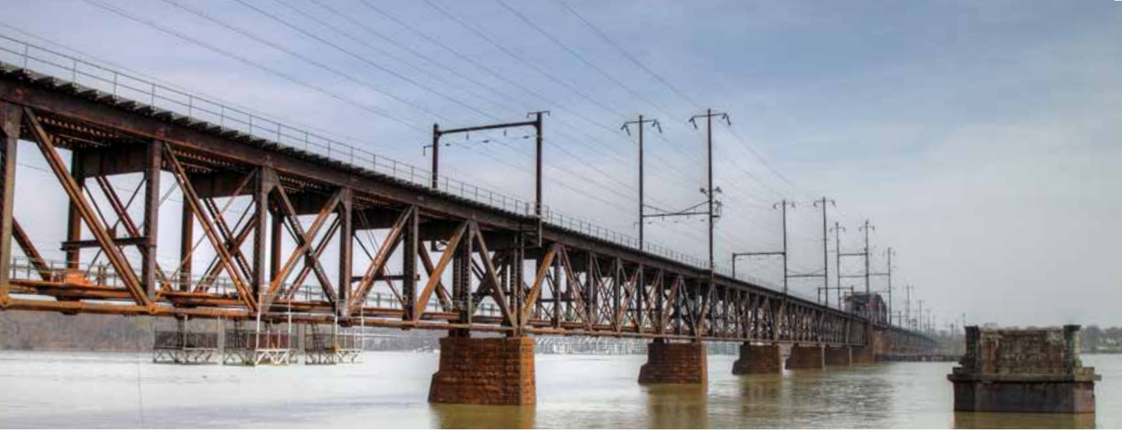
The Susquehanna River Bridge in Maryland
