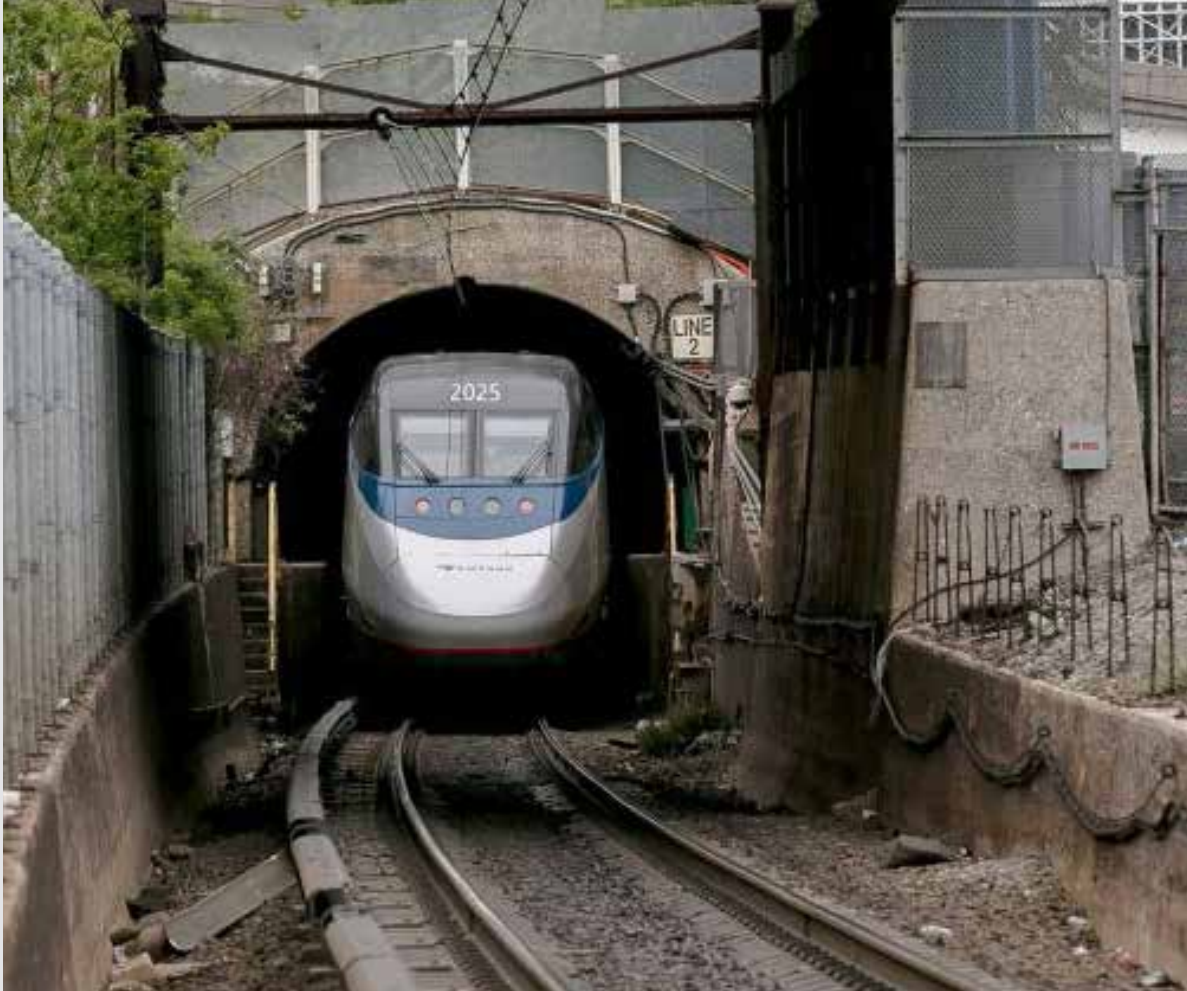
Amtrak Acela train exiting the East River Tunnel (NY)
