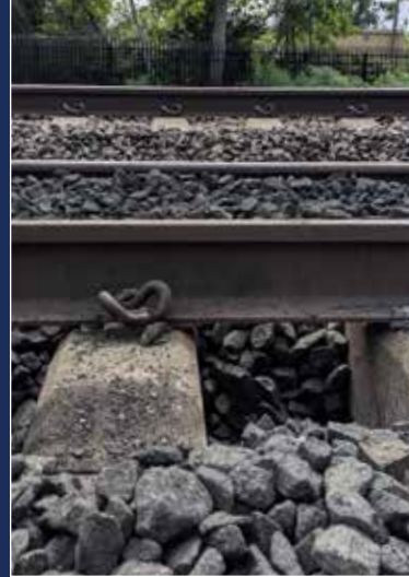
Starting from left to right: Crews operate the undercutter during a continuous outage near Canton, MD in August 2019. Middle: A view of track that sits on top of ballast, which helps with drainage and ensures proper alignment of the track. Right: Ballast over time erodes and becomes dirty with fouled material, shown here as the darker areas next to new, lighter-colored ballast.
