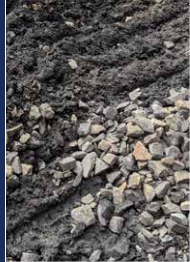
Starting from left to right: Crews operate the undercutter during a continuous outage near Canton, MD in August 2019. Middle: A view of track that sits on top of ballast, which helps with drainage and ensures proper alignment of the track. Right: Ballast over time erodes and becomes dirty with fouled material, shown here as the darker areas next to new, lighter-colored ballast.
