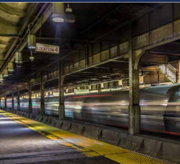
Newark Penn Station, shown above, is one of the busiest stations in New Jersey. The station serves over 27,000 and 1,000 NJ TRANSIT and Amtrak customers, respectively, each weekday.
