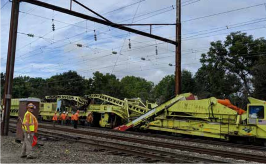
Starting from left to right: Crews operate the undercutter during a continuous outage near Canton, MD in August 2019. Middle: A view of track that sits on top of ballast, which helps with drainage and ensures proper alignment of the track. Right: Ballast over time erodes and becomes dirty with fouled material, shown here as the darker areas next to new, lighter-colored ballast.
